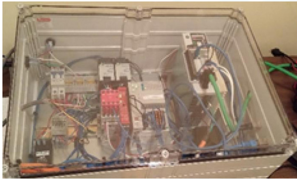
Figure 4: The electronic and electrical components, including the motor drive programmable controller (PLC), network adapter, and power supplies, were mounted inside a hard plastic enclosure. These components were connected to the motor via cables for motor power and control and operator interface.
